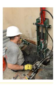
Once the resistance pier is connected to the bracket, adjustments with hand-held equipment will be made to lift and stabilize
